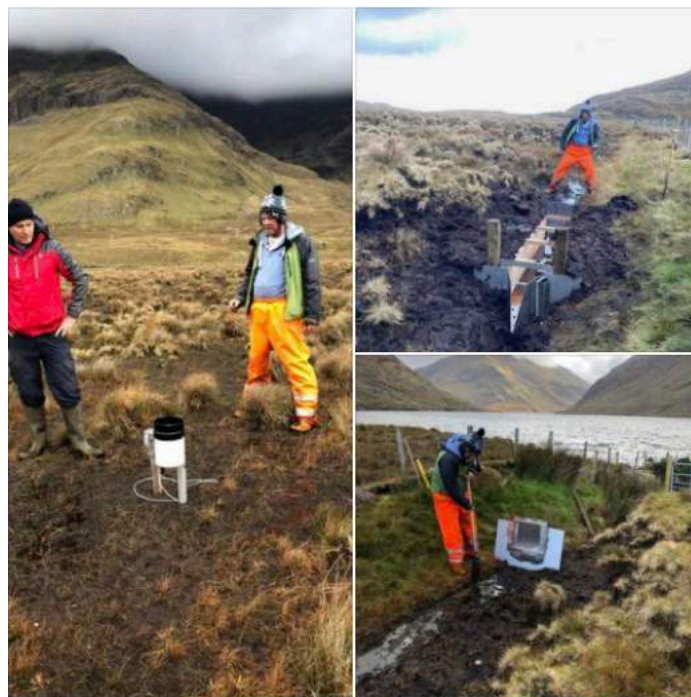
Figure 12. Flume and rain water gauge installation at Bundorragha commonage restoration site.
